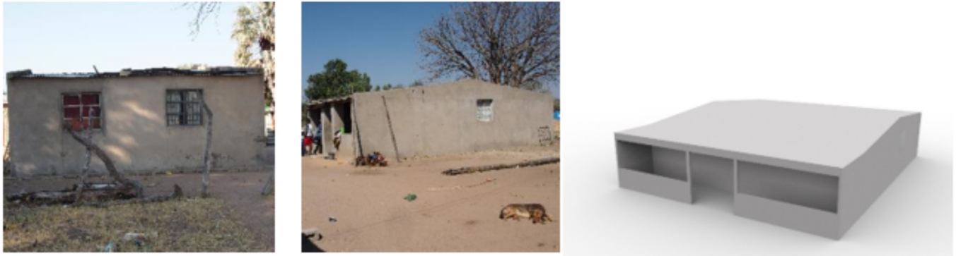
Fig. 6. House in Naipalala, Ondjiva. Composition of the walls: 2 cm of plaster + 12 cm of cement bricks + 2 cm of plaster. Composition of the roof: Corrugated zinc sheets.
