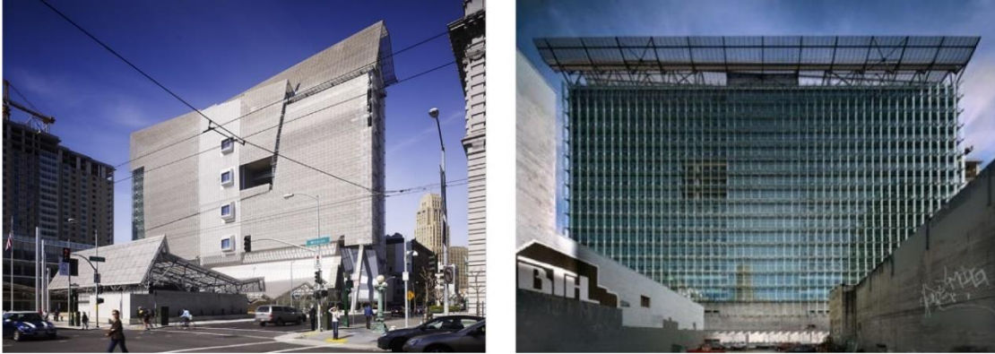
F9 – San Francisco Federal building's South façade with perforated metal as shade (left); North façade with vertical glass as brise-soleils.
